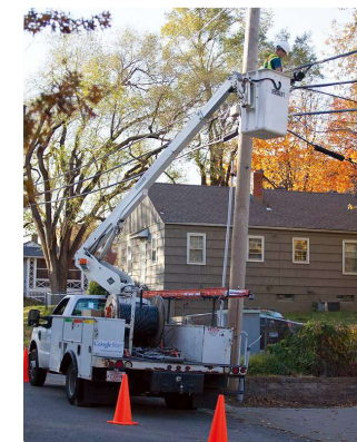
Outdoor Bucket Truck Installation
