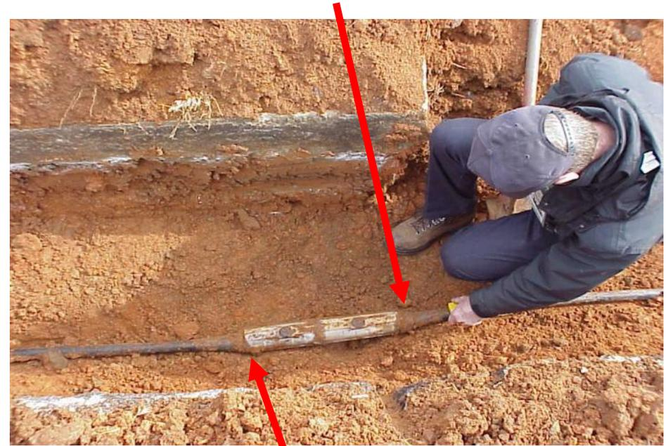
The Locate Tone was NOT present on the field side of the splice case indicating the open shield was in the splice case
